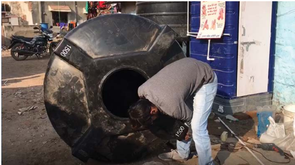
(Pictured: the extensive excavation required in install the bio-toilet tanks)
