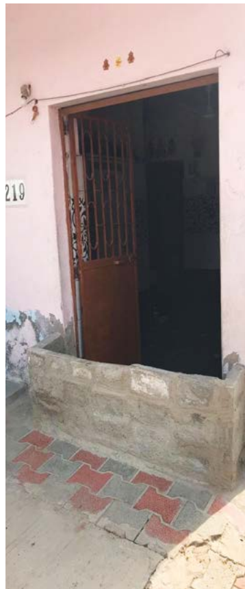
Fully constructed brick embankments at the entrance of houses.
