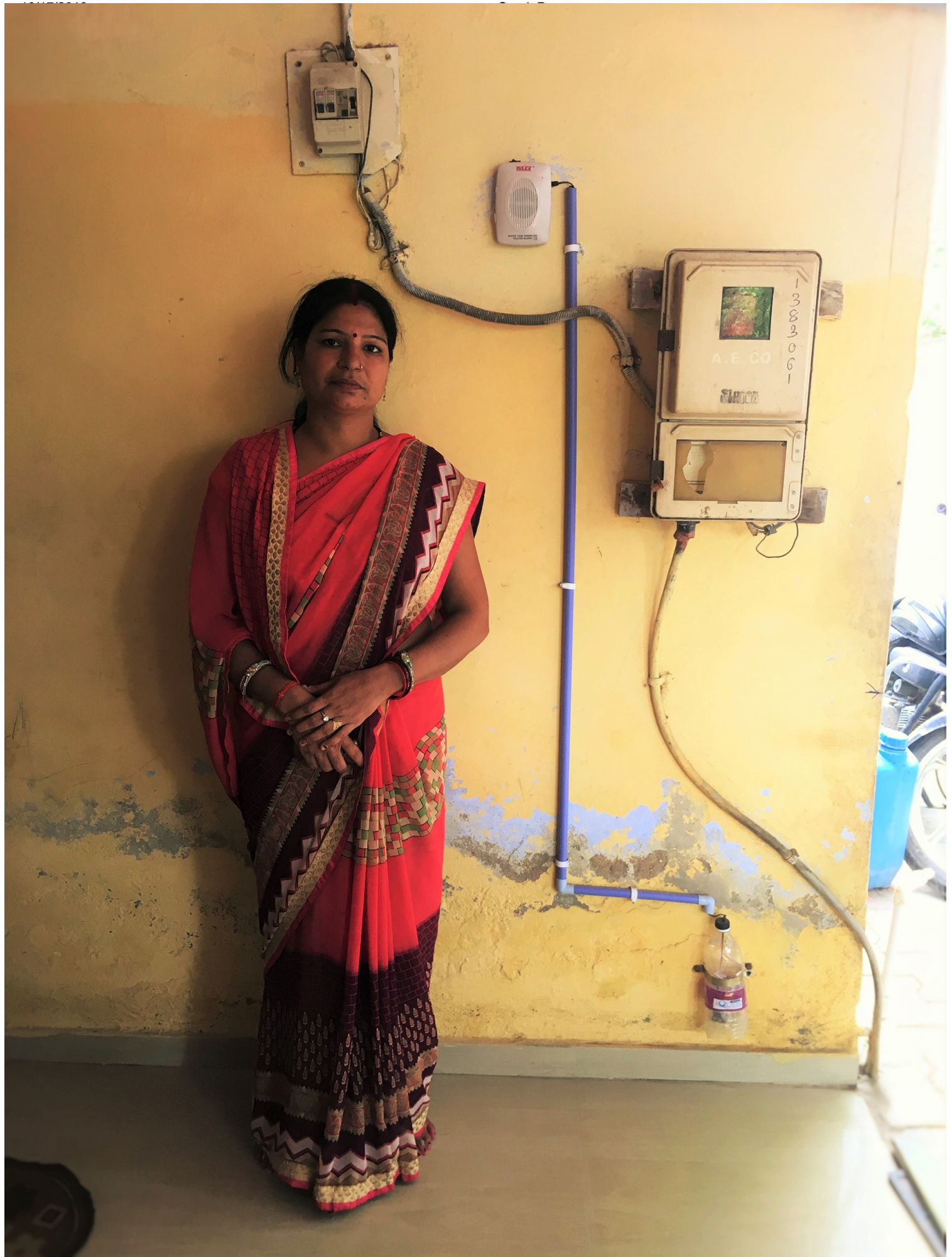
Radhika Ben showcasing the alarm installed by MHT in her house in Odhav.
