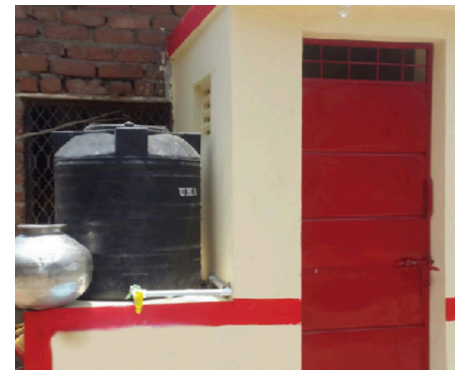
The toilet block constructed at Rekhaben's house.
