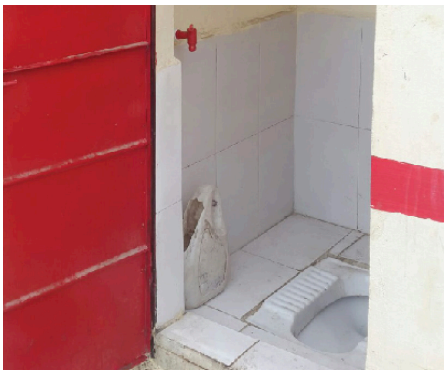
Inside the toilet is a ventilator, tap, and the SATO pan. The SATO pan looks similar to the normal pan.
