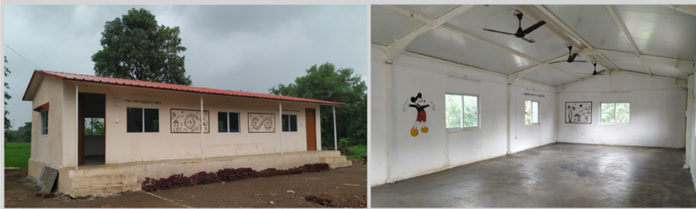
Post construction of the dining hall through prefabricated construction.
