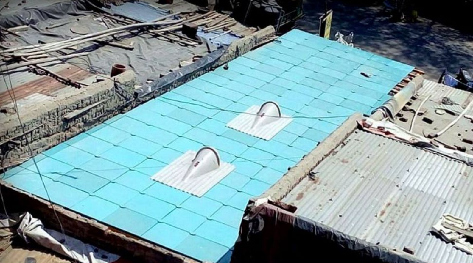
Modular roof with air lite ventilation.
